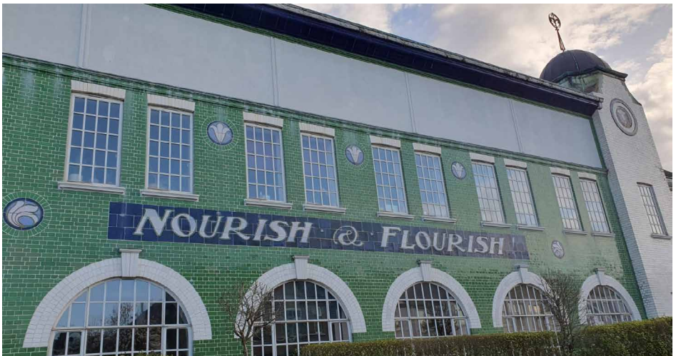
Former Frame Foods factory, Southfields, Christopher Arnsby, 2024
