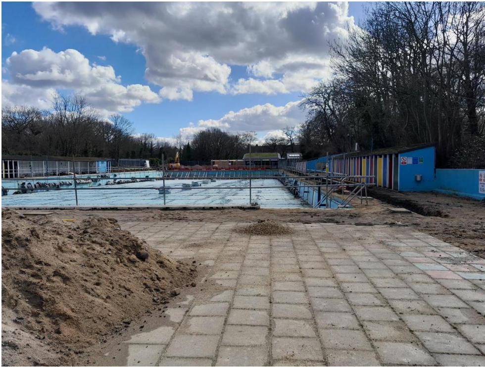
Photograph 1: Main pool and amenity space – u1b
