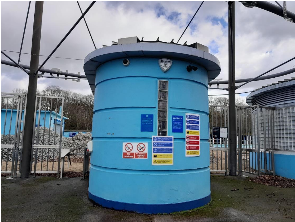
Photograph 7: Building B2 – u1b5
