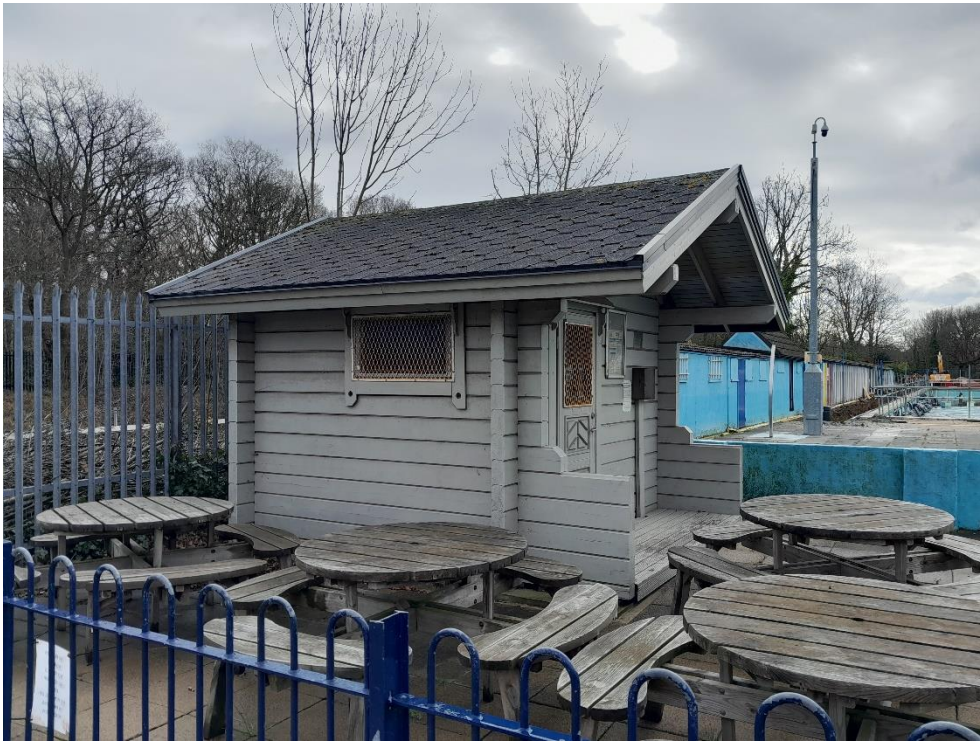
Photograph 9: Building B5 – u1b5
