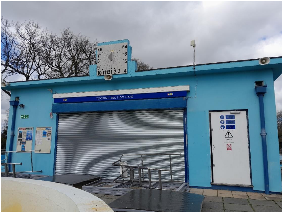
Photograph 6: Building B1 – u1b5
