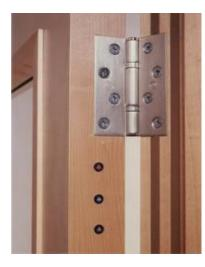
**Hinges** - A minimum of 3 fire rated hinges must be used with correct intumescent pads, location and fixings.
