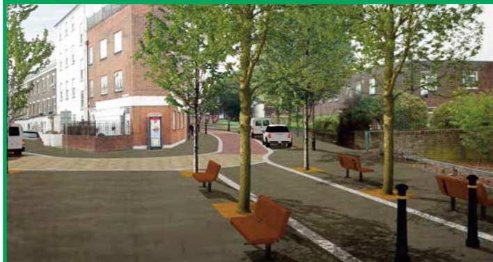
Figure 4 - After improvements: Junction with Simpson Street
