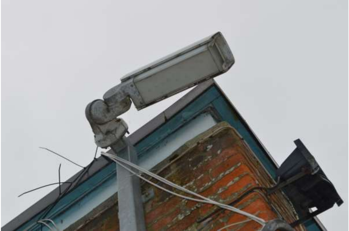
11: North-western corner of Northern Building showing the modern roof build up underside.
