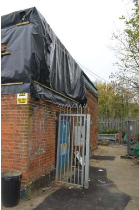
38: View looking north-east towards the southern elevation.
