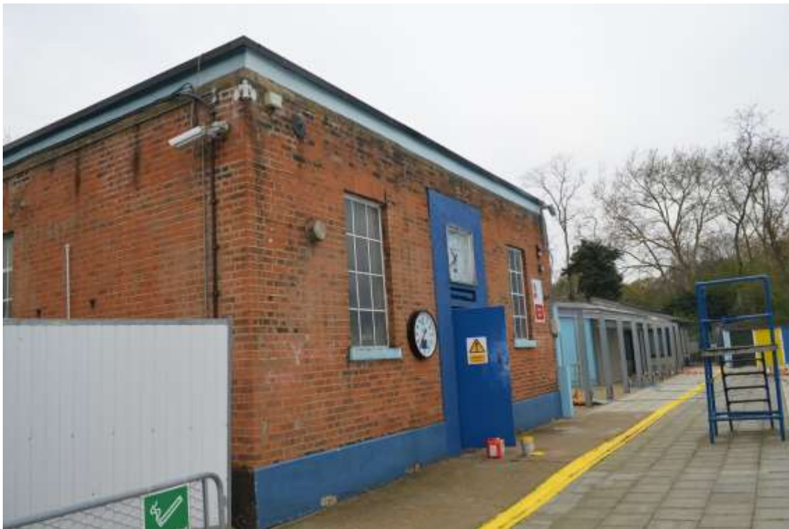
2: North-eastern corner of the North Building.
