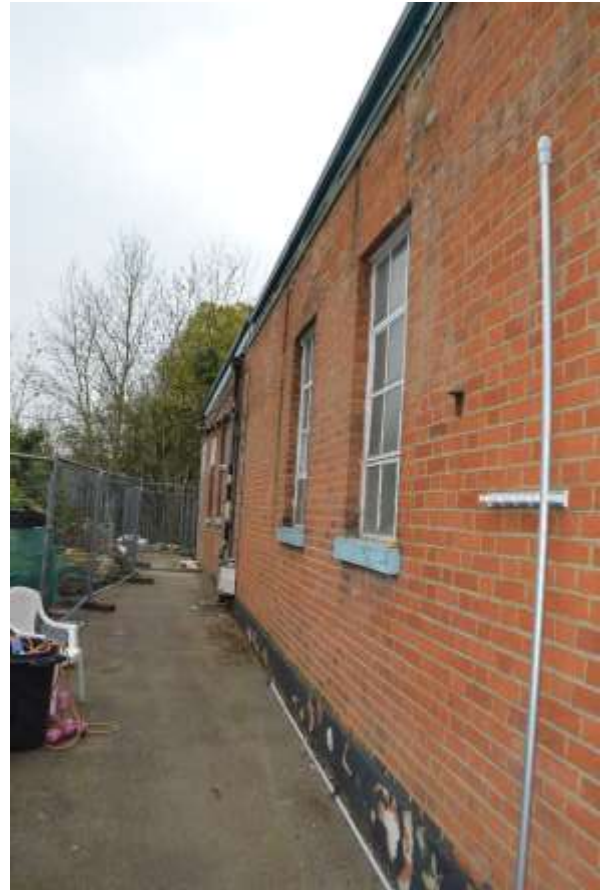
14: View looking south along eastern elevation towards the Southern Building.
