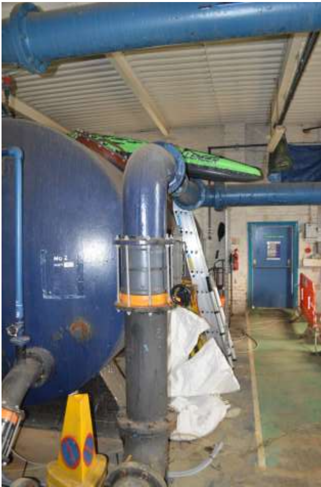
63: View looking south towards the southern elevation doorway.
