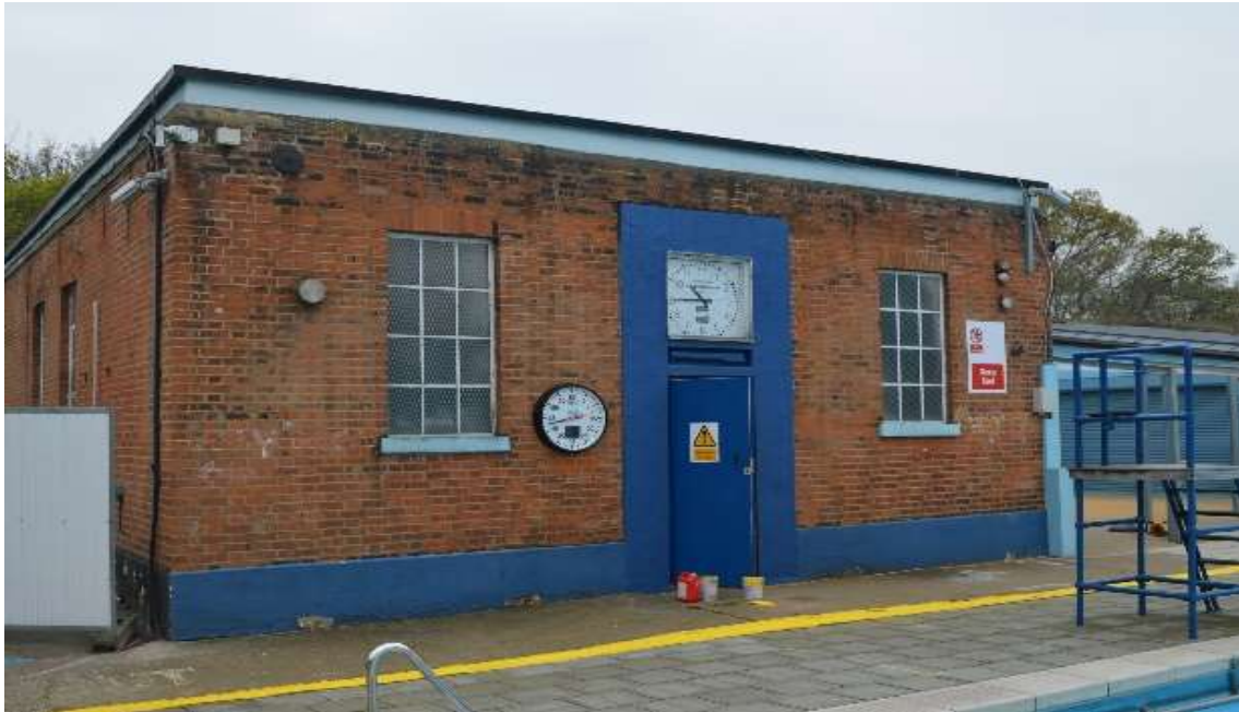
1: Northern elevation of Northern Building.
