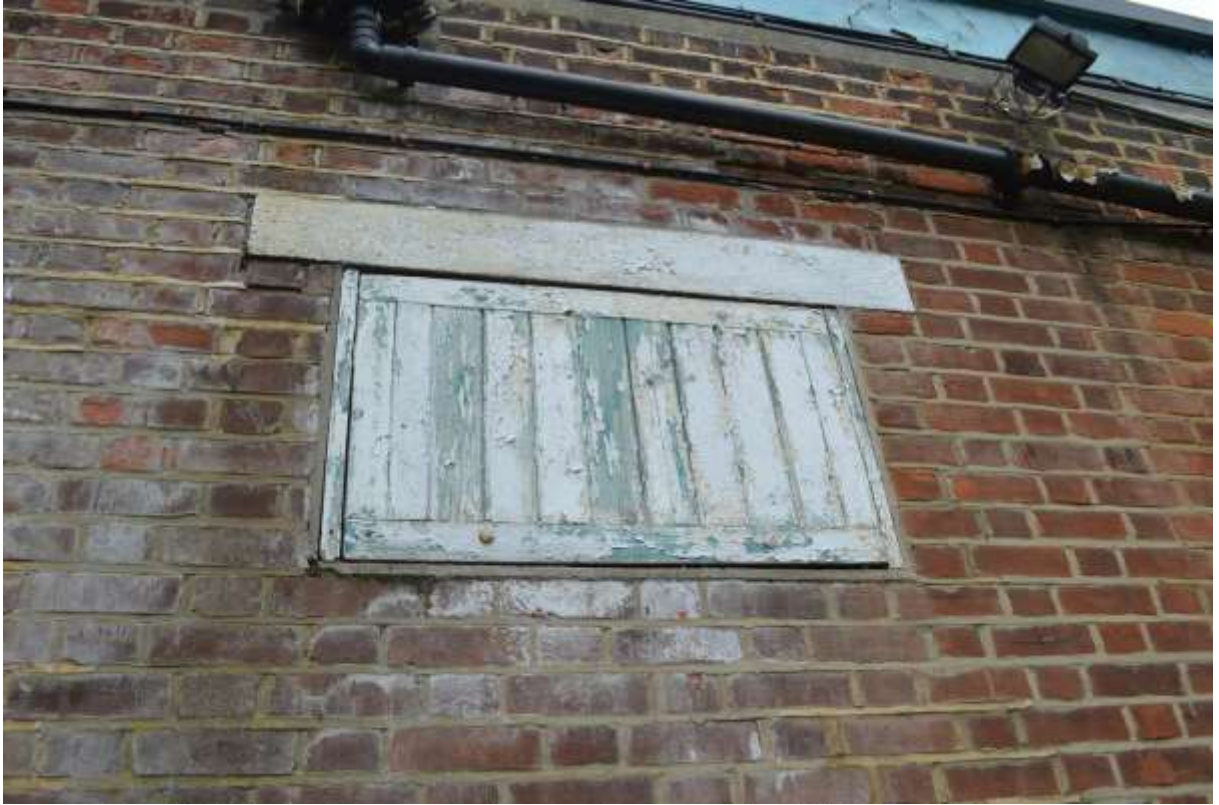
37: Most southern window on the eastern elevation.
