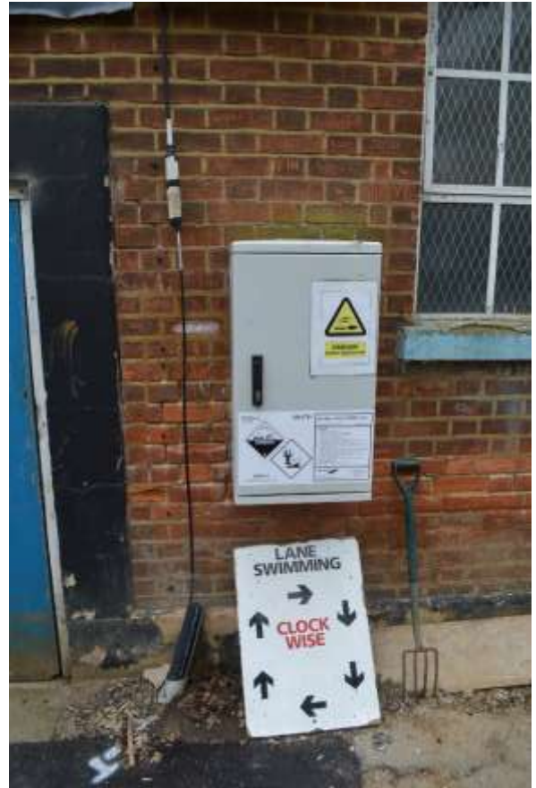
41: Modern chemical storage box on the southern elevation.
