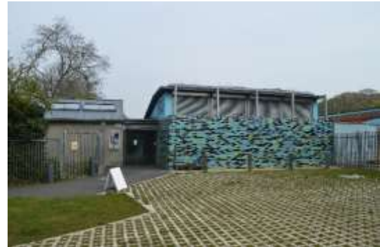
New pavilion building.
