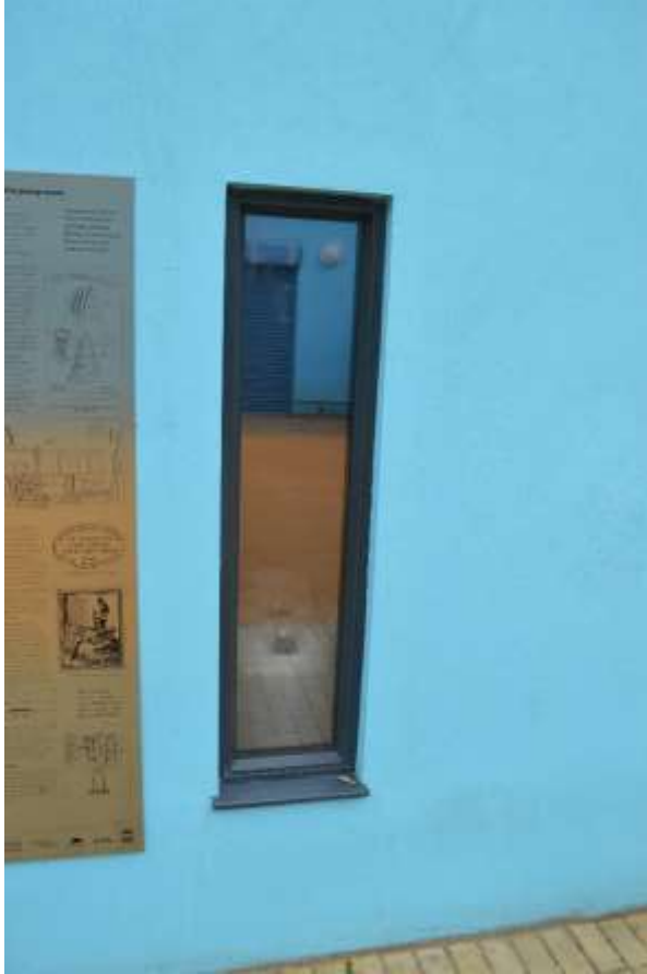
20: New window to western elevation.
