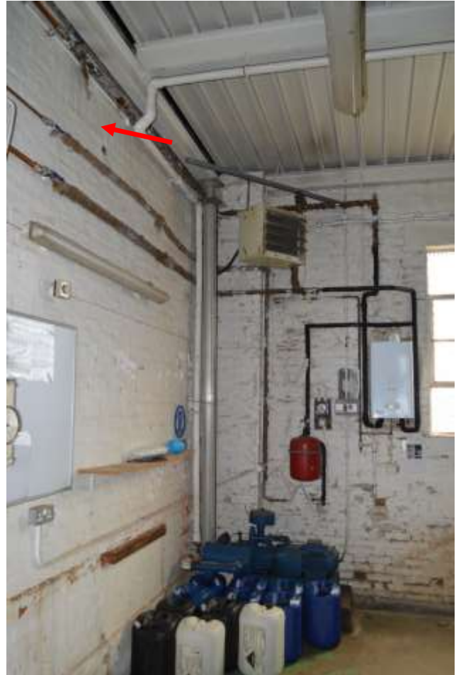
54: View of the north-eastern corner of the Southern Building. Note the former window lintel to the former southern elevation of the Northern Building marked in red.
