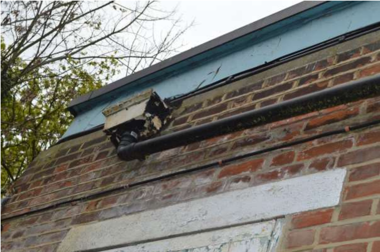
35: Cast iron hopper to the southern extreme of the eastern elevation.
