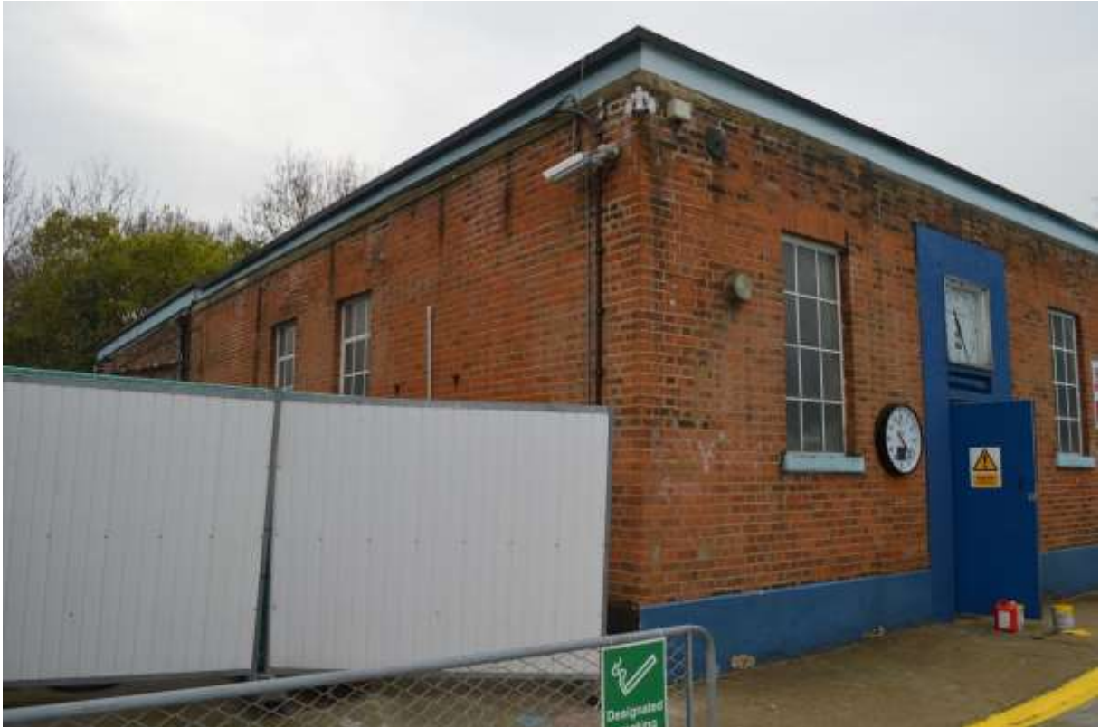
12: North-eastern corner of Northern Building showing the security camera to the northern end of the eastern elevation.
