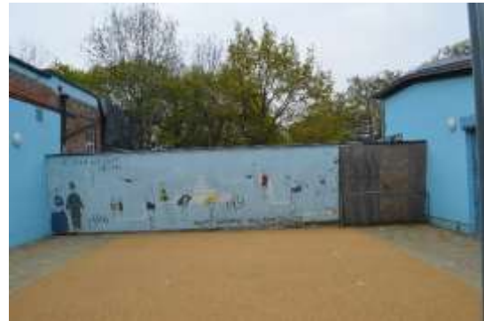
Location of the former entrance between the new pavilion and the Pump Room.
