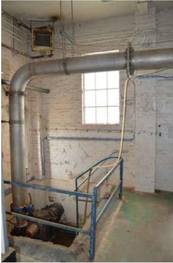
22: Small lower ground floor area to north-western corner.
