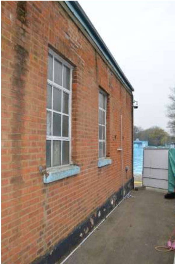
13: View looking north along eastern elevation towards the pool.
