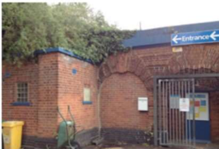
Figure 5.19: The entrance arches prior to demolition, southern elevation.
