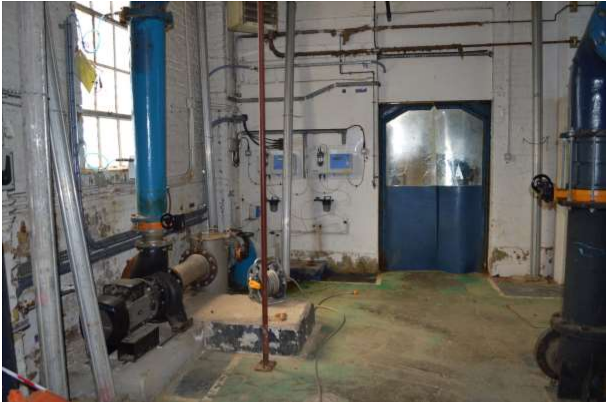
65: View of the north-western corner of the Southern Building.
