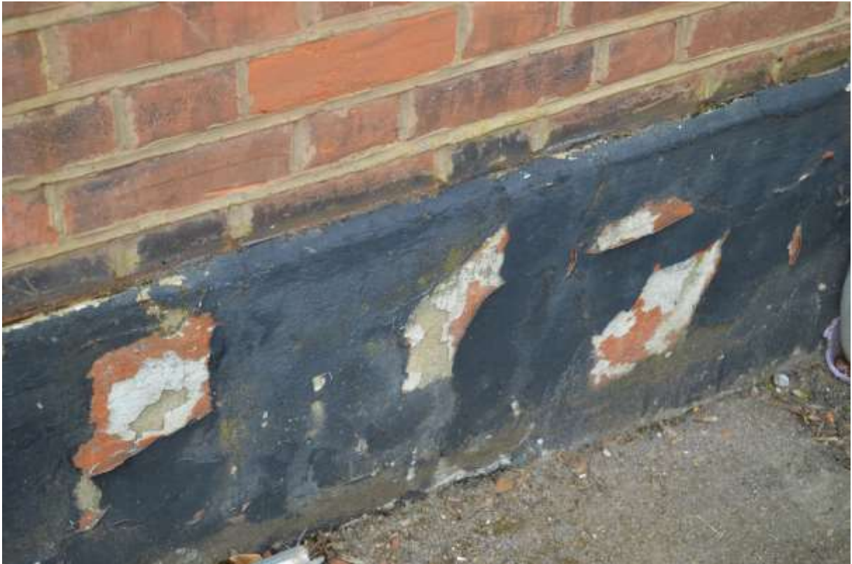
16: Cementitious rendered plinth at low level.
