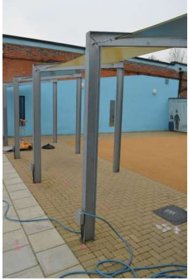
21: New covered walkway adjacent to western elevation.
