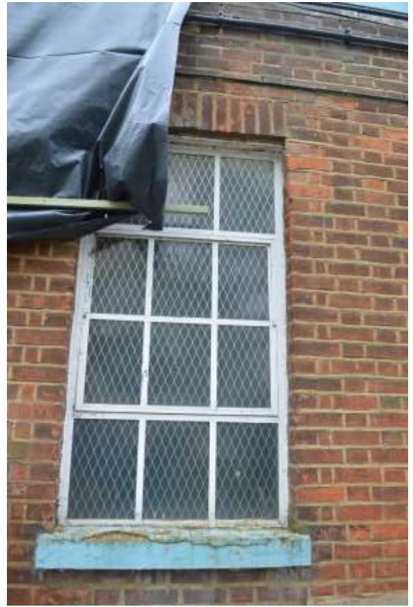
39: Steel framed window on southern elevation with central pivoting panes.
