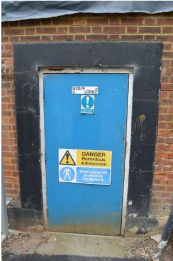
42: Door to southern elevation with cementitious render architrave.
