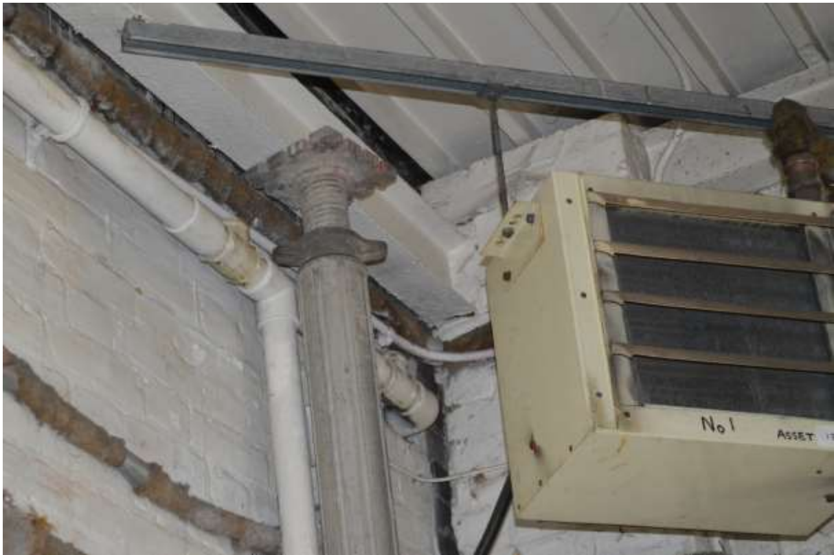
55: Showing the modern roof above and a close up of one of the temporary Acrow props.
