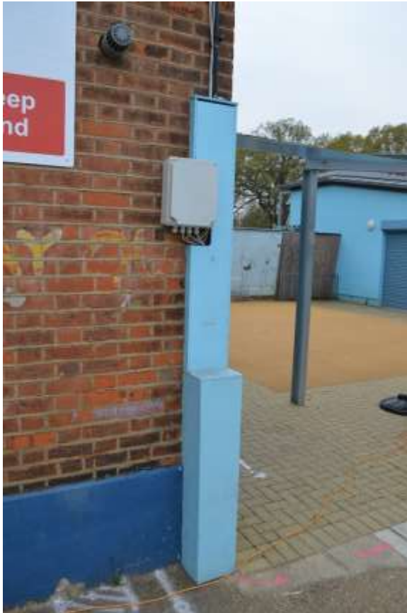
9: Riser to north-western corner of Northern Building.
