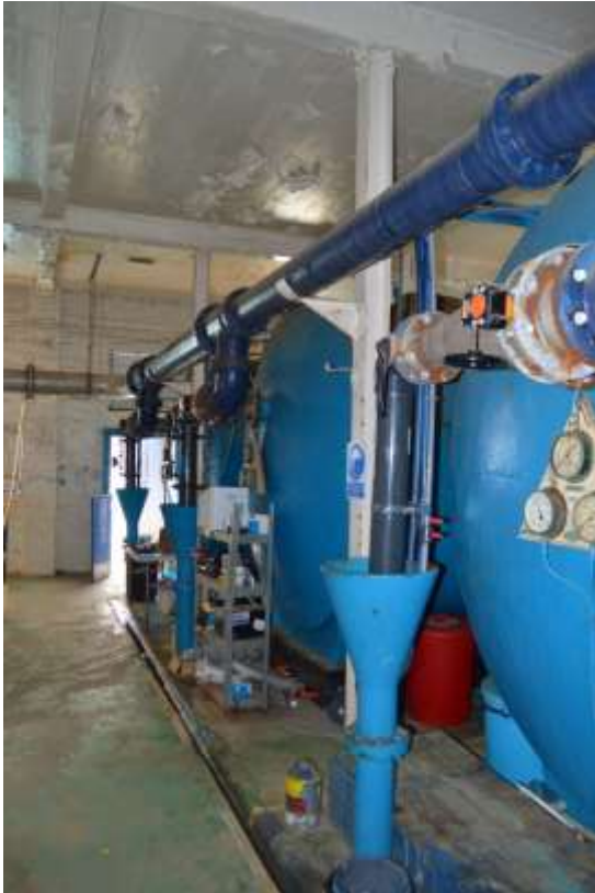
27: View looking north-east showing cylinder outlets Nos 1-3.
