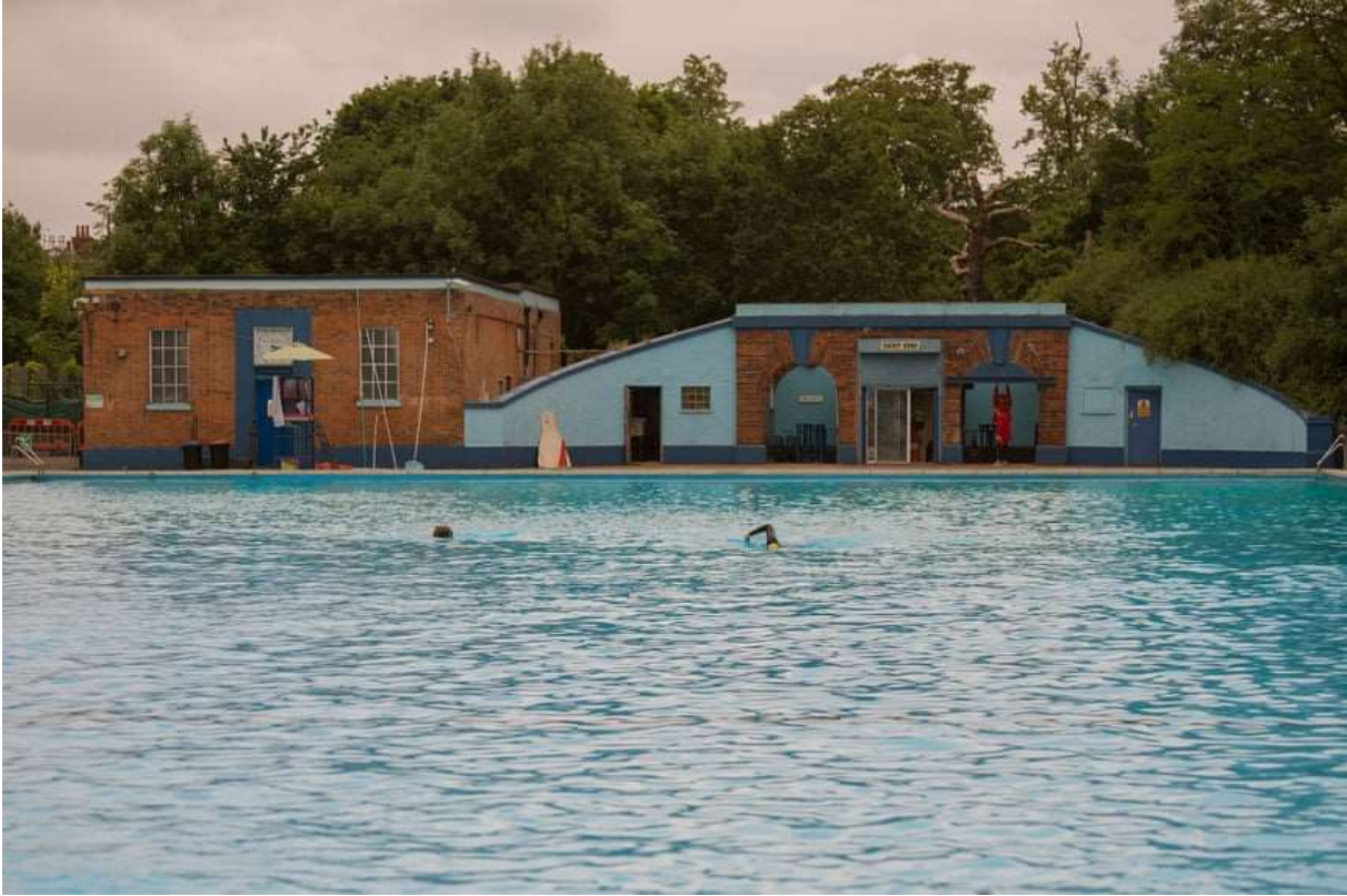
Figure 5.20: The entrance arches prior to demolition, northern elevation.
