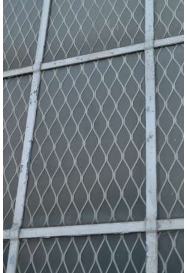
6: Steel framed window with glazing bar loops.
