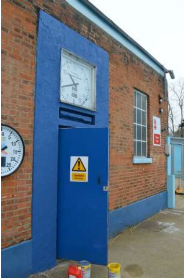
7: Showing main entrance door to front elevation, render architrave detail around door and clock and central clock above doorway.
