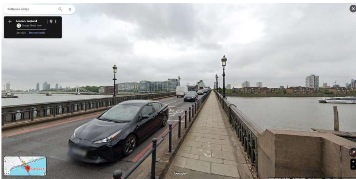
Fig 1. Image looking towards application site from the north side of Battersea Bridge (Source: Google Street View)
