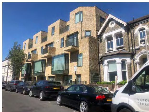
Fig. 363: 4-8 Hafer Road scheme photo
