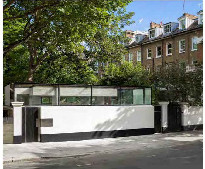
Fig.339: Earl's court house - A contemporary design on a small site that discreetly slots into a conservation area.
