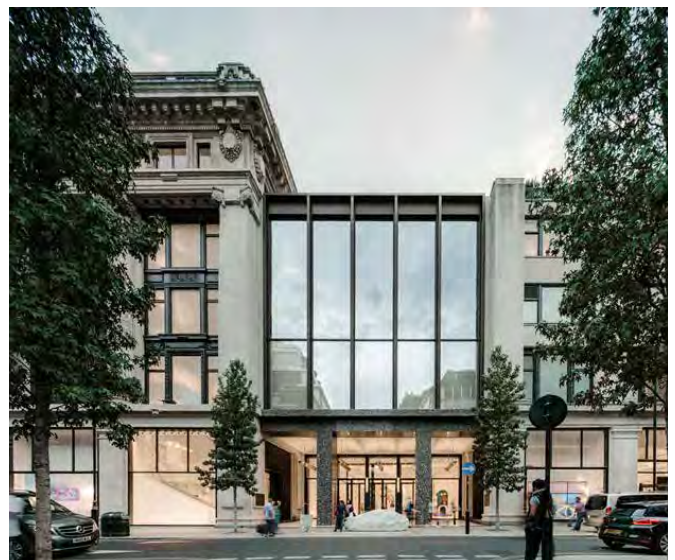
Fig.338: Selfridges, Duke street - The new addition respects existing massing and materials while incorporating a contemporary architectural character.
