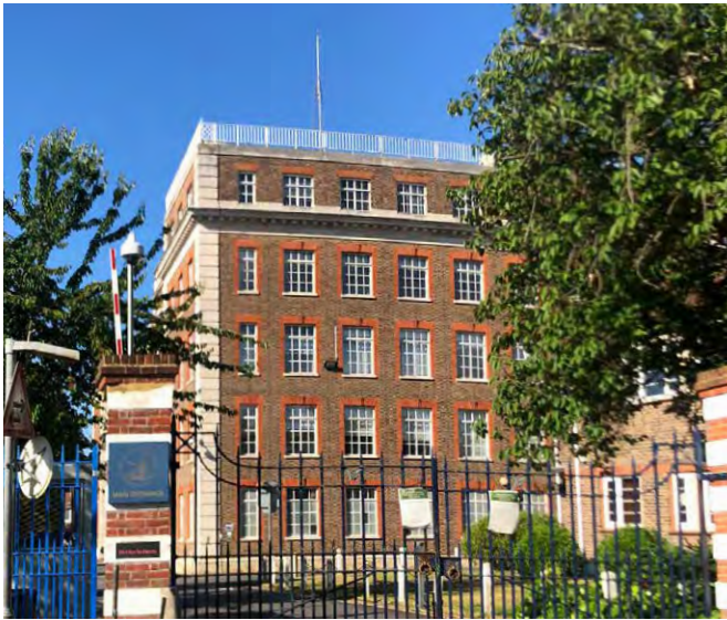
Fig.177: Red brick imposing 5 storey building of the Bank of England Sports Centre
