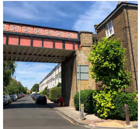
Fig.161: Railway bridge at Fawe Park Road
