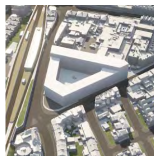
Fig. 242: Sainsbury's car park, Bedford Hill
