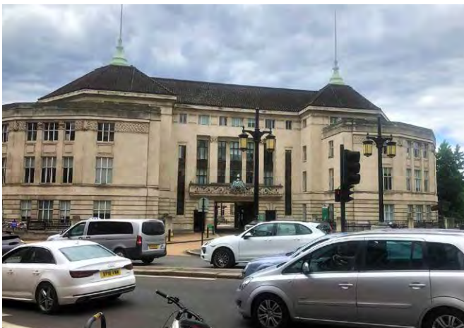
Fig. 394: Wandsworth town hall
