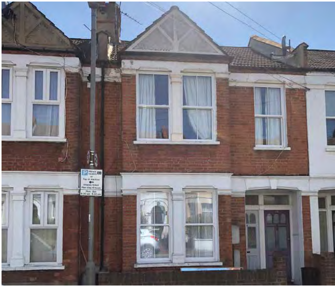
Fig. 197: Two storey period terraces on Totterdown Street
