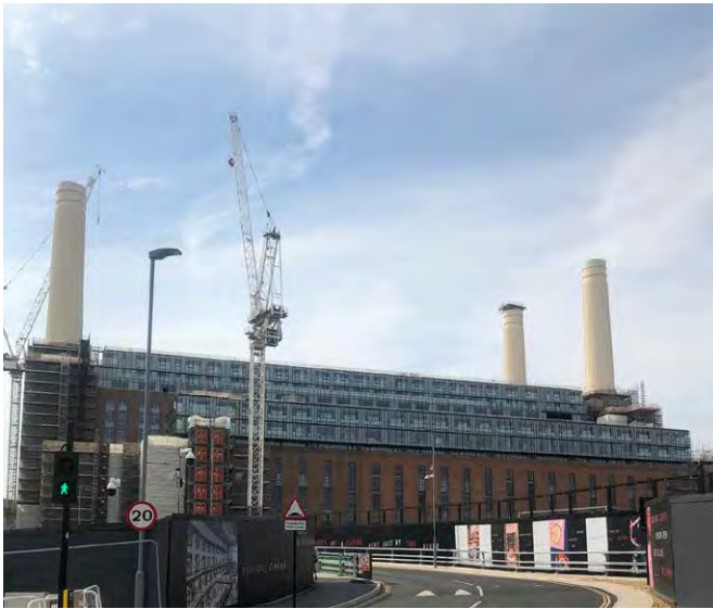
Fig. 93: The iconic Battersea Power Station during redevelopment
