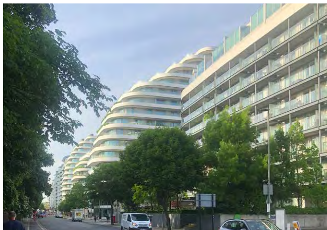
Fig.383: High-rise flats in Nine Elms
