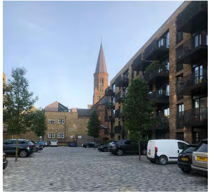
Fig.301: This new development in Granfield Street successfully responds to the nearby Grade II Church of the Sacred Heart in Battersea Square Conservation Area, through use of high quality bricks, and use of subtly different coloured bands of bricks. Successful use of sensitive architectural detailing and its subservient scale to the church landmark, alongside the courtyard space which frames views to the spire.
