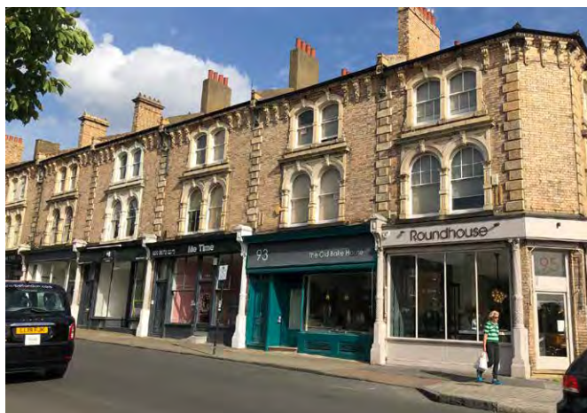
Fig.385: Shop front terraces in Balham
