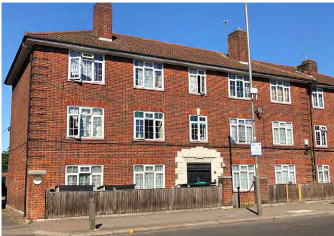
Fig. 378: Low-rise flats house in Tooting
