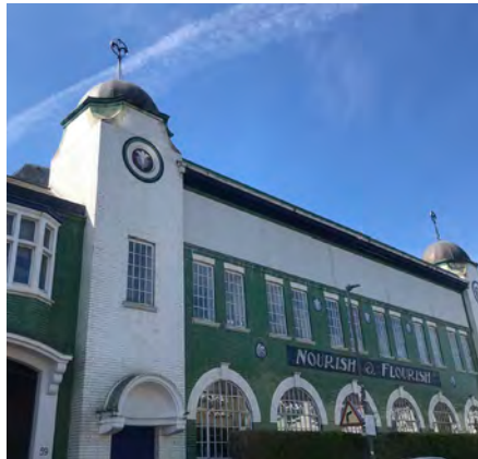
Fig.110: The distinctive ceramic tiled factory of Frame Foods (grade II listed), now converted into flats
