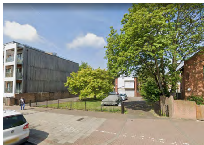
Fig.444: Rectory Lane small sites existing site
