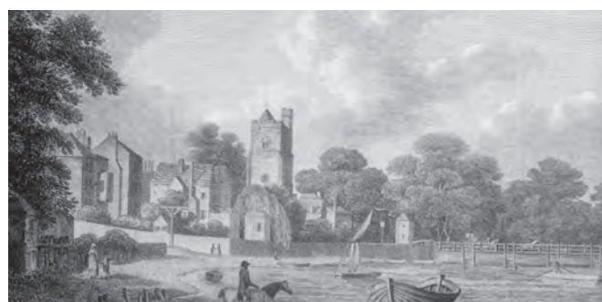
Fig.11: View upstream along the river bank from Old Putney Bridge, 1796
