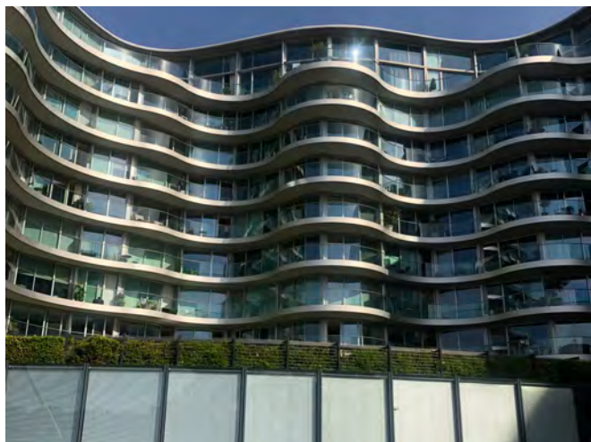
Fig. 282: Albion Riverside building
