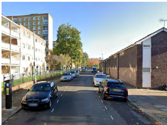
Fig. 263: Existing 4 and 11 storey blocks on Blondel Street
