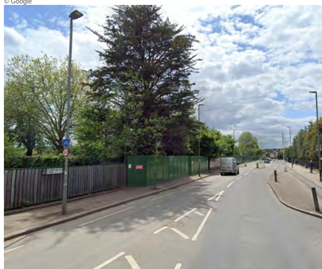
Fig.554: Burntwood Lane looking south west Photo © Google
