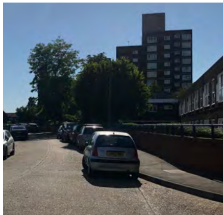
Fig.162: Low-rise and high-rise estates at Arabella Drive
