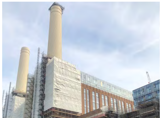
Fig. 286: Battersea Power Station undergoing redevelopment
