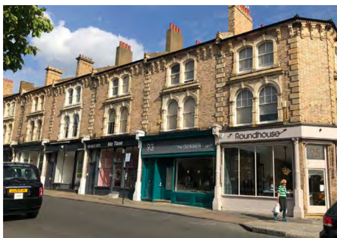
Fig. 497: Shopfront terraces in Balham
