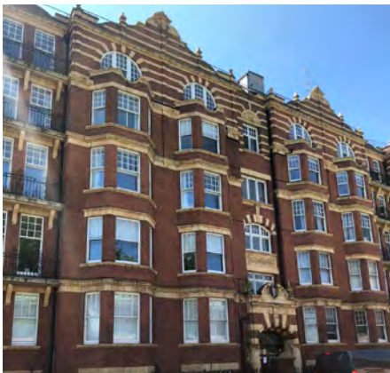
Fig.129: Kenilworth Court mansion blocks with views across Putney Bridge and the river
