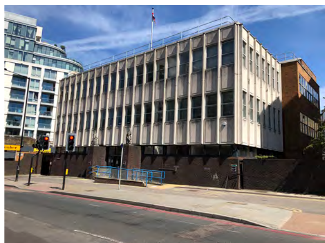
Fig. 344: Between the railway line and Woodlands Way
