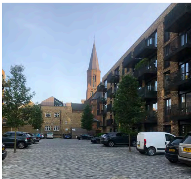
Fig.414: This new development in Granfield Street successfully responds to the nearby Grade II Church of the Sacred Heart in Battersea Square Conservation Area, through use of high quality bricks, and use of subtly different coloured bands of bricks. Successful use of sensitive architectural detailing and its subservient scale to the church landmark, alongside the courtyard space which frames views to the spire.
