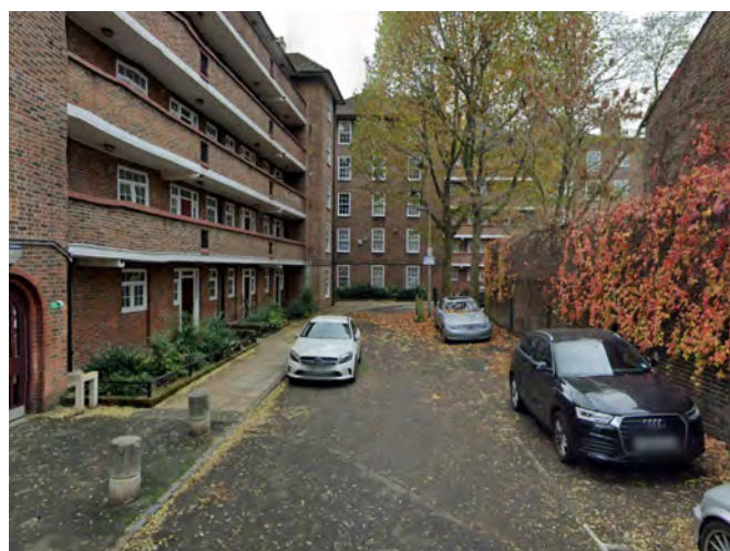
Fig.289: 5 storey blocks on Savona Street
