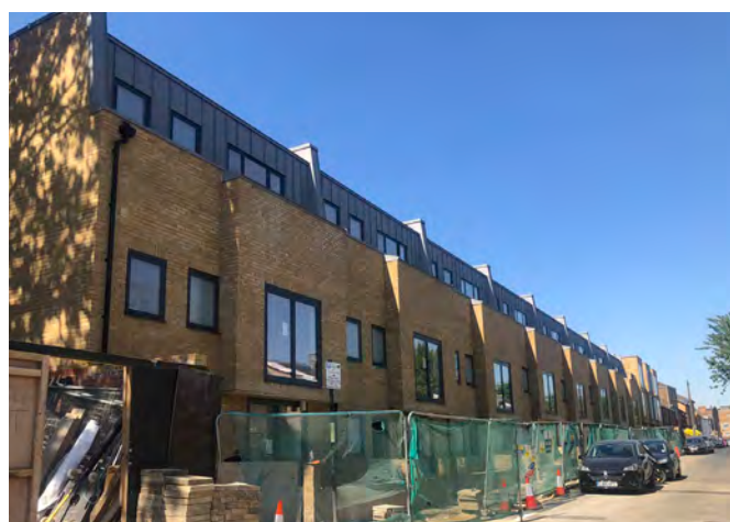
Fig.430: Precedent new build terrace row along Balham New Road
