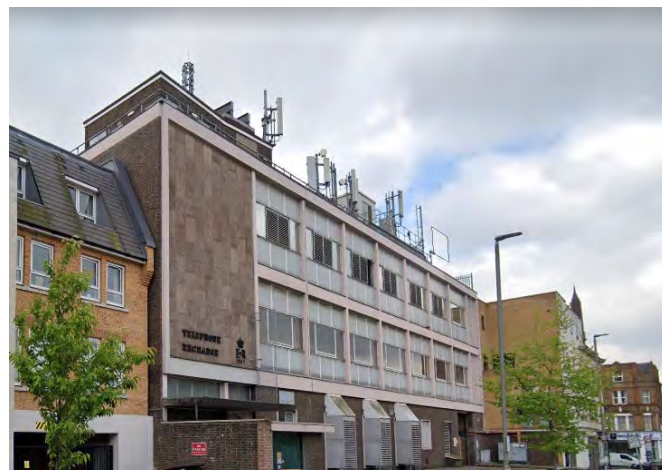
Fig. 437: Old Telephone Exchange small sites existing site
