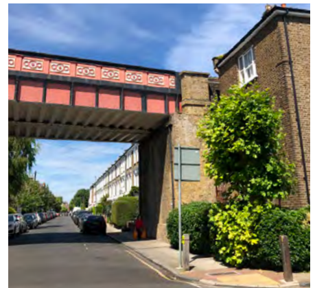
Fig. 143: Railway bridge at Fawe Park Road
