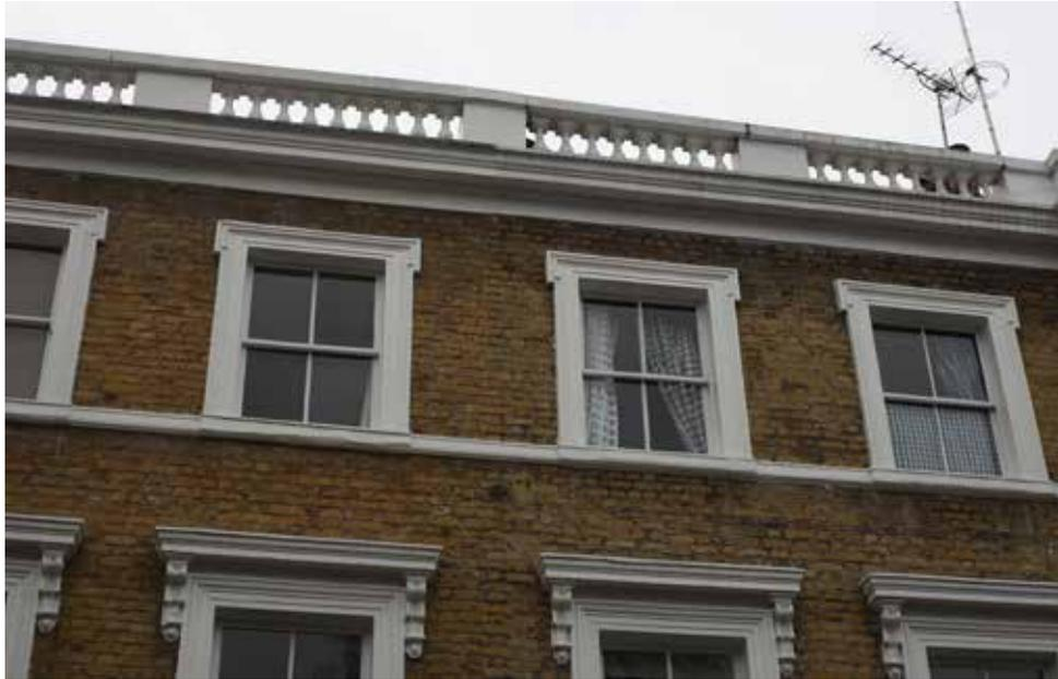
Parapet roofline with stucco cornice and balustrade concealing a butterfly roof behind, Margaretta Terrace
