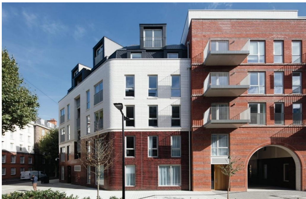
Figure A1.1 Bourne Estate – An example of a linear block residential type
