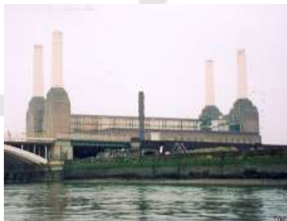
Battersea Power Station decommissioned
