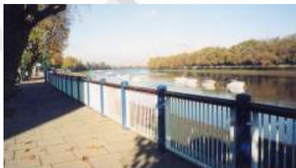
Balustrade Putney Embankment
