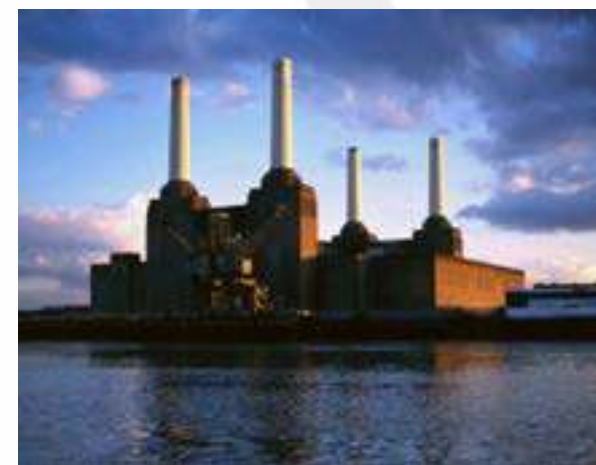
Sir Giles Gilbert Scott's Battersea Power Station
