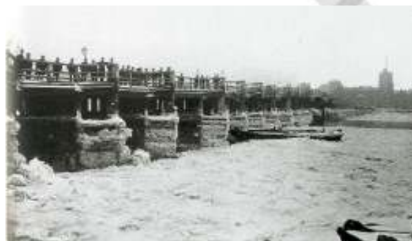
Old Fulham Bridge, 1881
