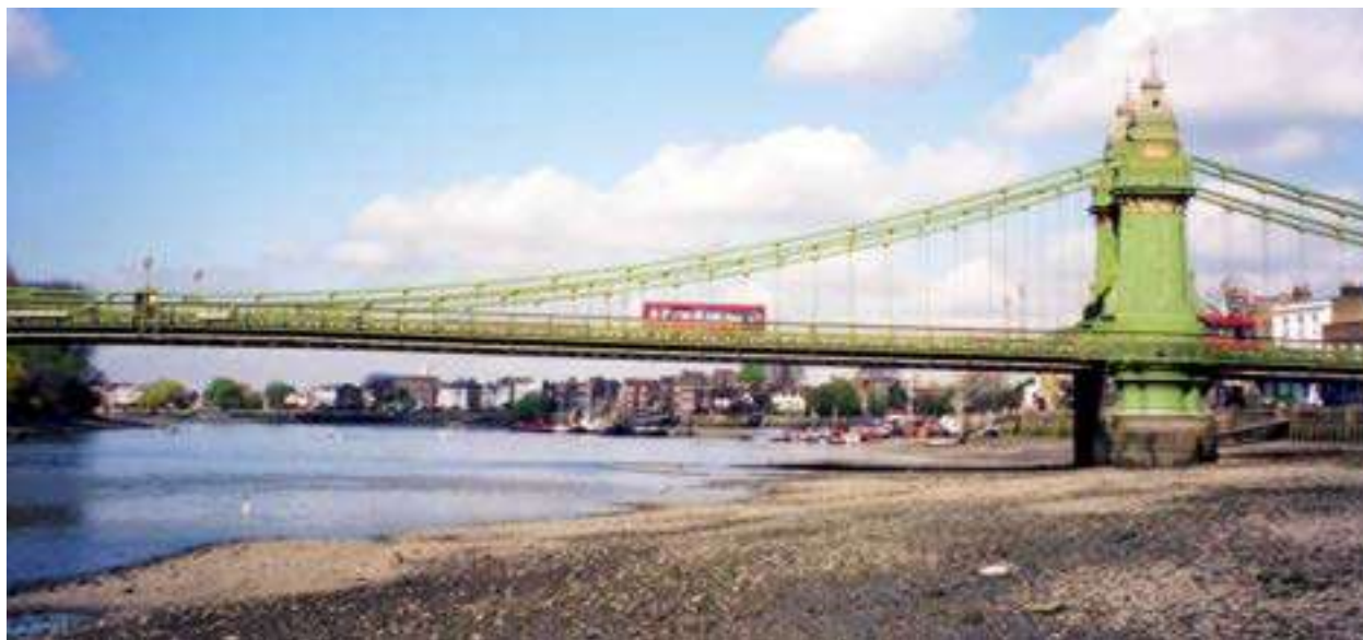
Hammersmith Bridge looking upstream
