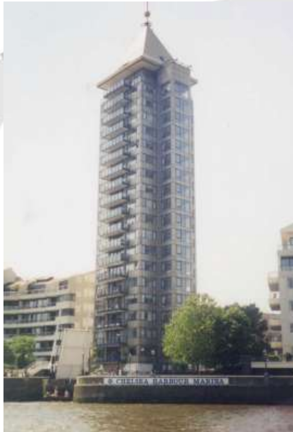
Belvedere Tower, Chelsea Tower
