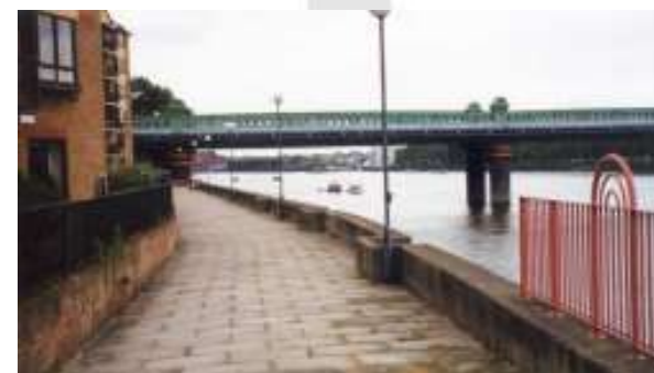
Fulham, above Putney Rail Bridge ~ Poor setting
