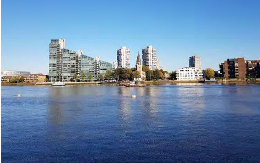
Fig. 87: St Mary's Church nestled among competing landmark buildings on Battersea Riverside including towers in Battersea Residential
