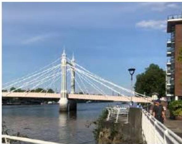
Fig. 73: View from the riverside promenade looking downstream to the listed Albert Bridge
