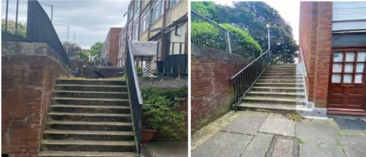
Steep level changes between Roehampton Lane and Harbridge Avenue requires a variety of steps to access homes at Kingsclere Close.
