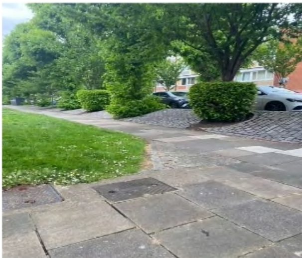
Steep level change between the pavement /road on the south side of Harbridge Avenue with no access points
