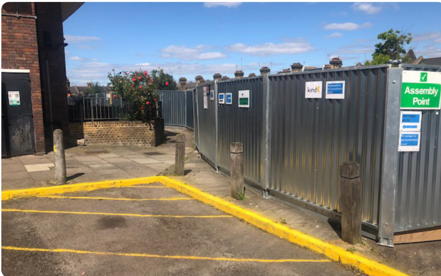
Reserved emergency vehicle parking location
